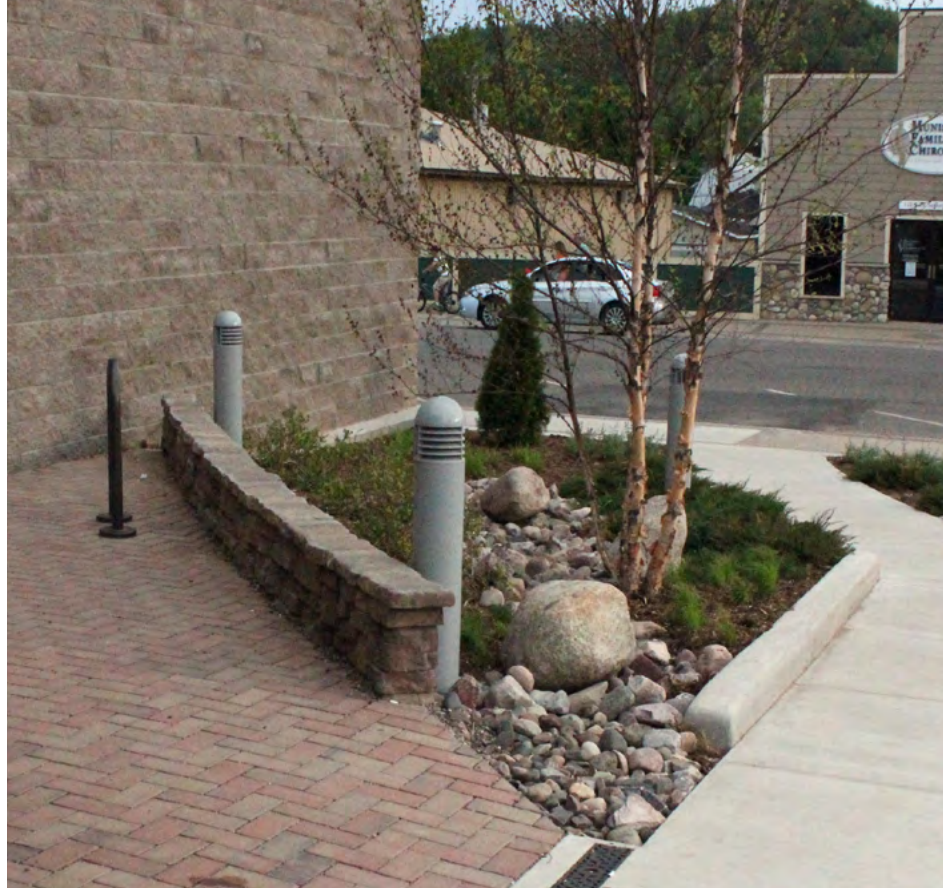
FIGURE 9.3 - Bus Stop In Munising Converted To Utilize Porous Pavement With A Rain Garden
